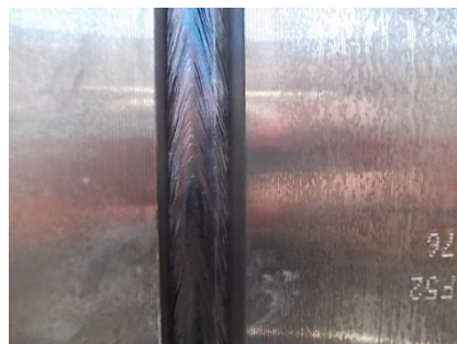
in progress Weld layers details
