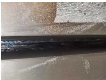
Interpass temperature check
